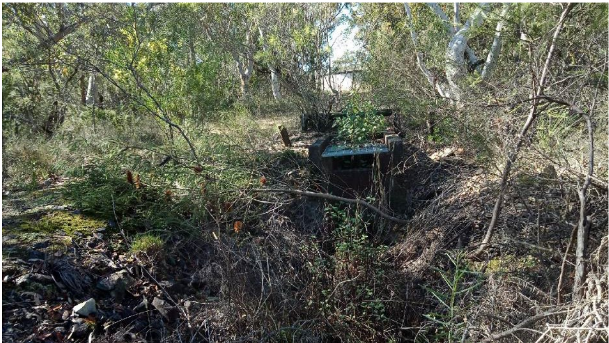
Plate 14: Drainage Channel cut north of WWR4
